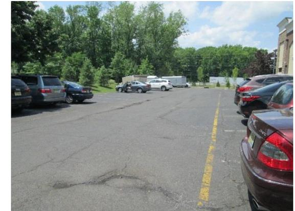
A rain garden can be installed north of the church to capture, treat, and infiltrate parking lot runoff. Parking spaces west of the building can be replaced with porous asphalt to infiltrate stormwater. A preliminary soil assessment suggests that more soil testing would be required before determining the soil's suitability for green infrastructure.
